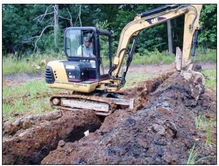
system and treated using an **Aquafix** system provided to the SRWC by the **US Department of Energy**. Prior to the stirring, a trench was dug lengthwise in order to examine the treatment media. Various distinguishable layers could be viewed including pockets (lenses) of limestone aggregate and decomposed compost material. Photos were taken and samples of the various layers were collected for analysis. Keep your eyes open for updates on the system in future issues of the Catalyst.
