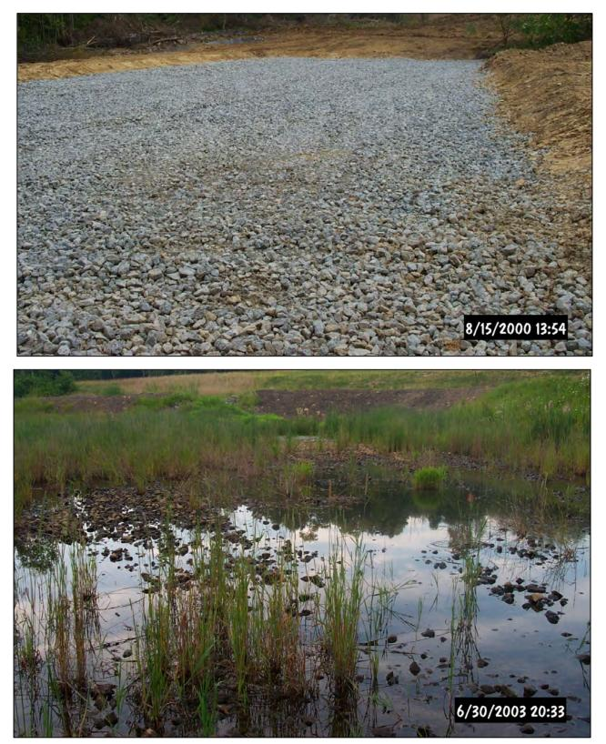
**De Sale Restoration Phase 2 Horizontal Flow Bed:** 2,900 tons of AASHTO #1 limestone (>90%CaCO<sub>3</sub>) shortly after construction (top). After about three years, reduced hydraulic conductivity caused water to flow across the top of the limestone treatment media (bottom) during seasonally high-flow periods.
