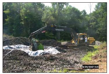
Figure 4. Excavator with FlipScreen attachment "washing" Mn covered limestone
